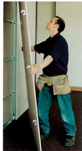
Removing panel from wall
